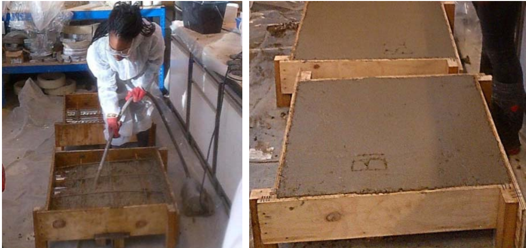
Figure 9 Concrete being cast and finished slabs
