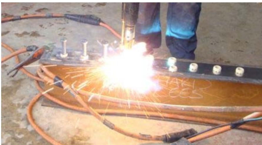
Figure 2 Through-deck welding trial
